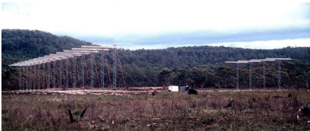
Figure 1.5: The 16 element transmitting and receiving array (left), and the four element interferometer receiving array (right).
